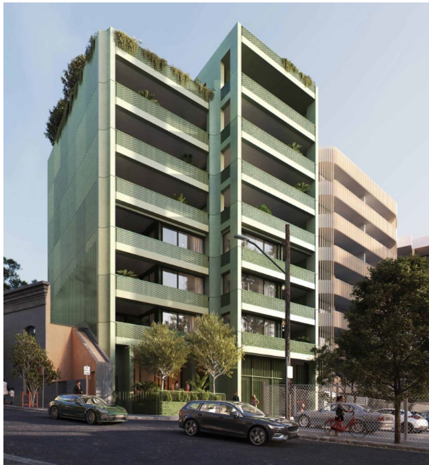
Holt Street looking south-west
